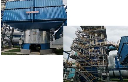
Heating and power generation system adopting RTO technology for ultra-low concentration coal mine gas(1% to 1.2%).
